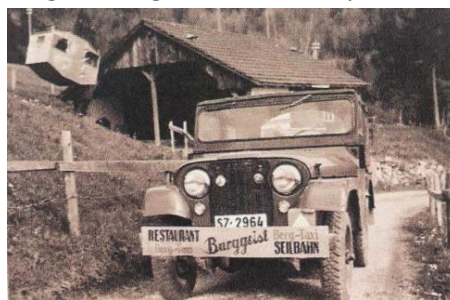
Transportseilbahn Feissenboden – Rigi Burggeist
